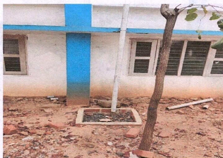
Rain Water Recharge Well
